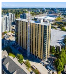
Brock Commons, Vancouver, [7]
