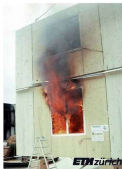
Non combustible surface in fire room
